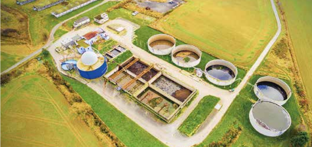
Biogas Plant 沼氣廠
