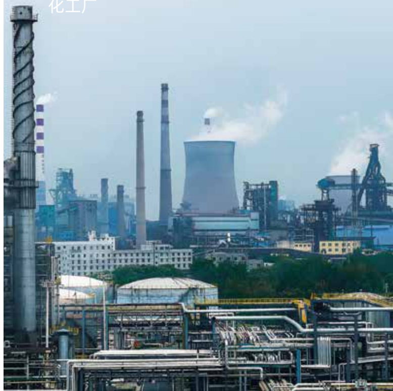
Chemical plant 化工厂
